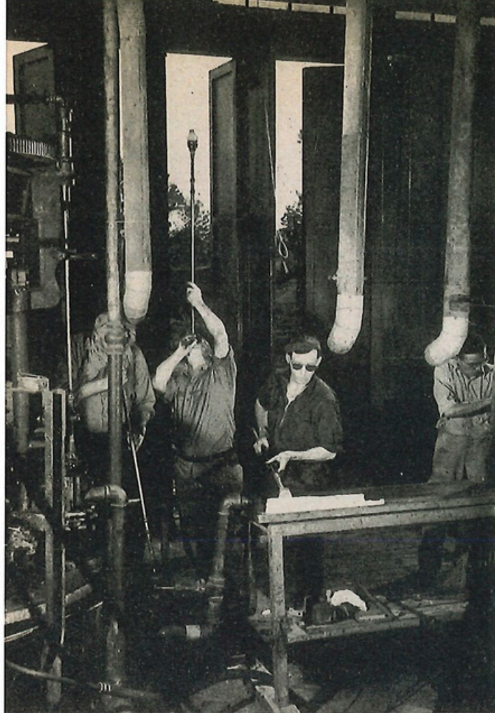
Glass blowing at the Aladdin plant, one of the few places in the United States where the old-fashioned method is still used for certain purposes. Most of these blowers are of Swedish descent.
