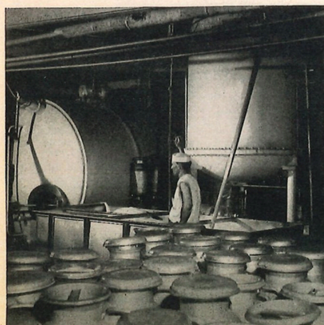
Feeding milk into a condenser, the first step in dehydration. The milk is then dried, rolled, and powdered. Dehydration reduces weight 90 per cent.
