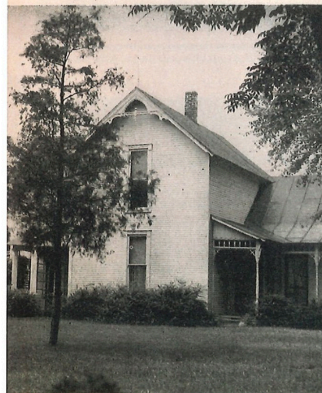
Water from the well, tested regularly for purity, is piped to the kitchen sink, but there is no other inside plumbing. Telephone lines will not be extended to the Blake neighborhood until after the war.
